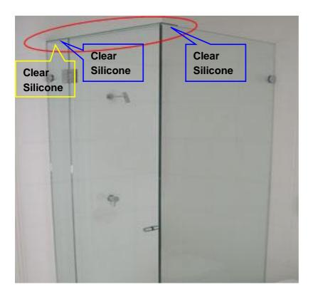
Step 12: (Optional) Place the glass corner shelve to the right height as shown in the photo below and mark a position for the wall mounting bracket. Repeat Step 3, slide the glass shelve into the bracket and tighten the grab screw with the screw facing down. Fill the gaps with clear silicone.
